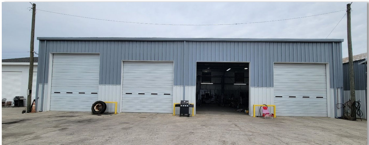
Figure 7. Duplin County Maintenance Garage
