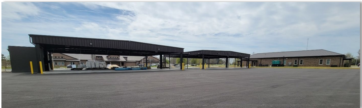
Figure 4. DCPT Covered Fleet Parking
